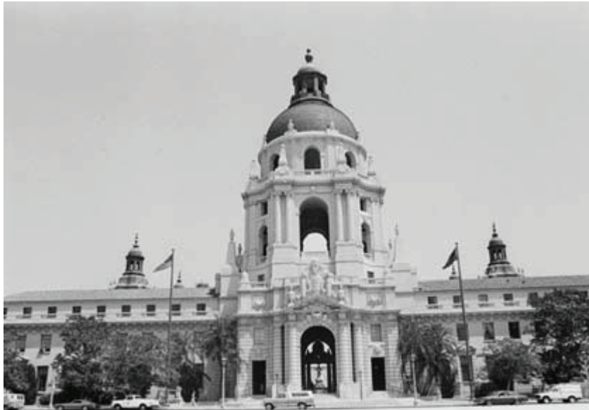
Pasadena City Hall, designed by Arthur Brown Jr., 1928. Photograph Courtesy of The Bancroft Library. BANC PIC 1981.161
